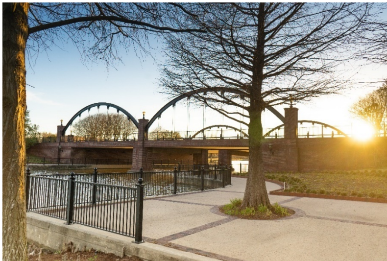
University Drive bridge in Sugar Land
