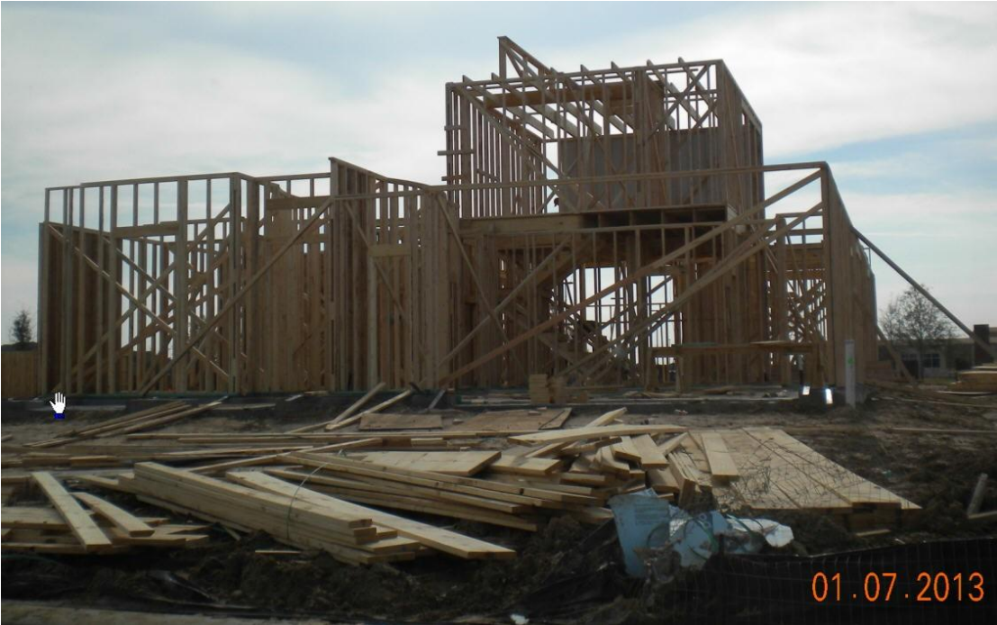
10% Framing started but not complete.
